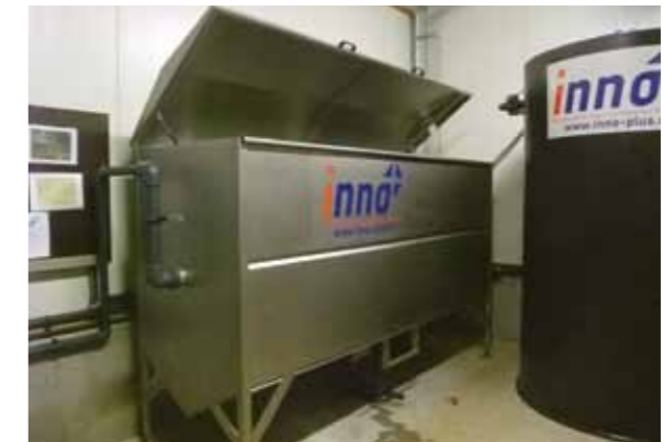
Inno+ Clean water sedimentation tank + denitrification reactor
