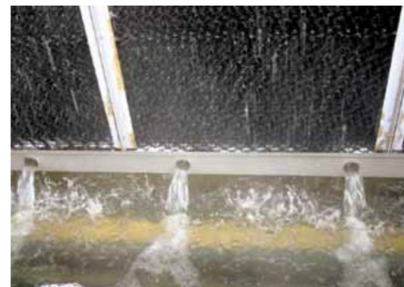
Scrubber filter after cleaning
