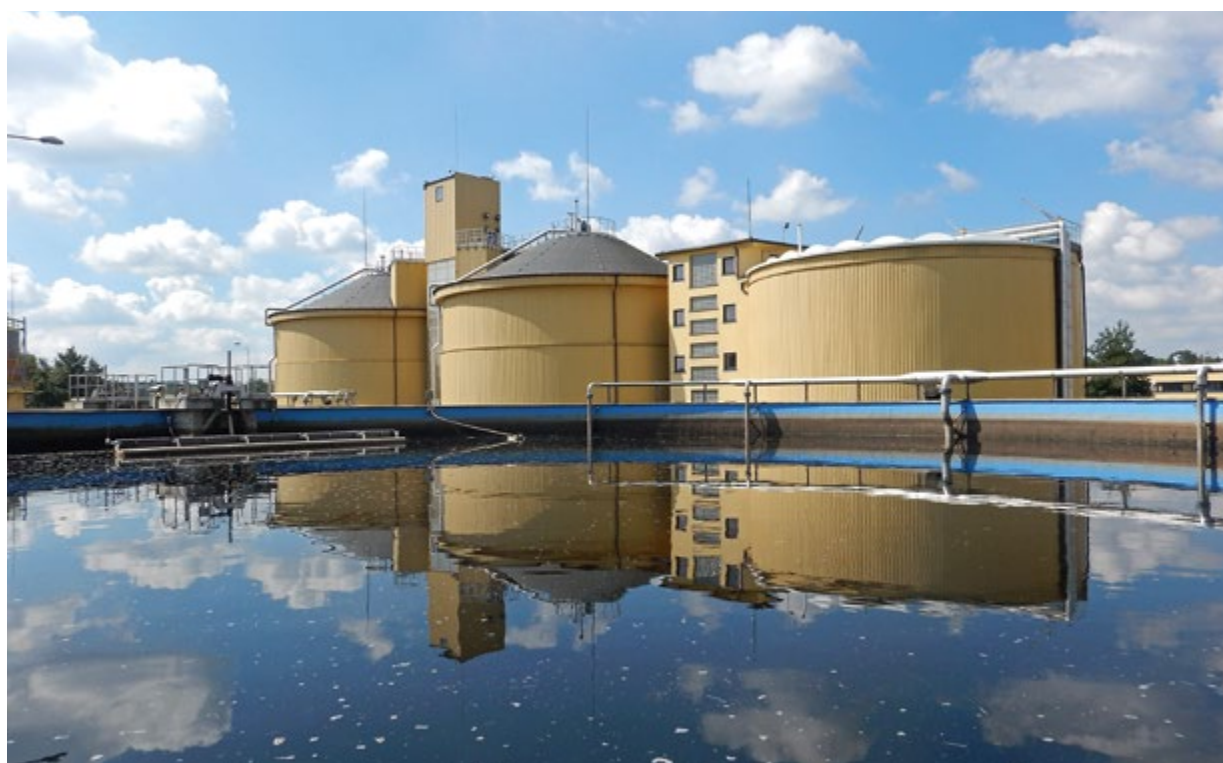
Photo 2. Digesters (2x5500 m 3 )
