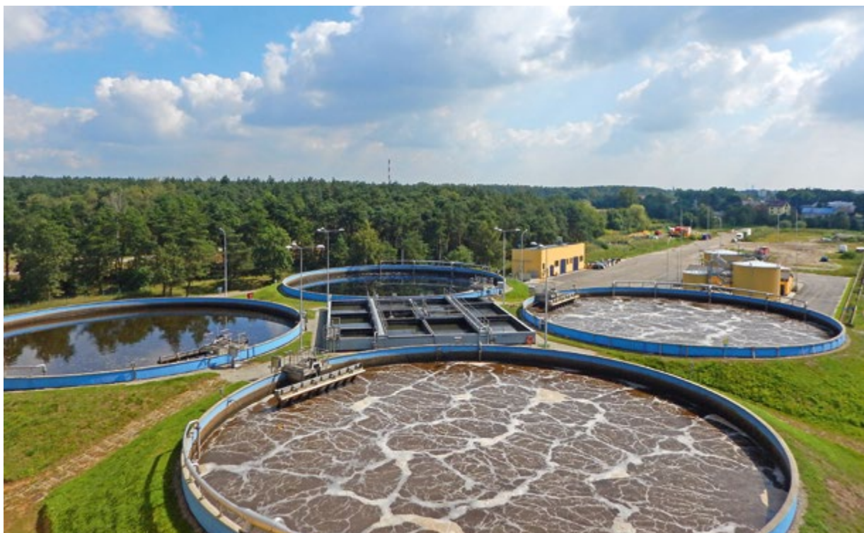
Photo 1. Modernised biological part of the plant - C-TECH Technology sequenced chamber
